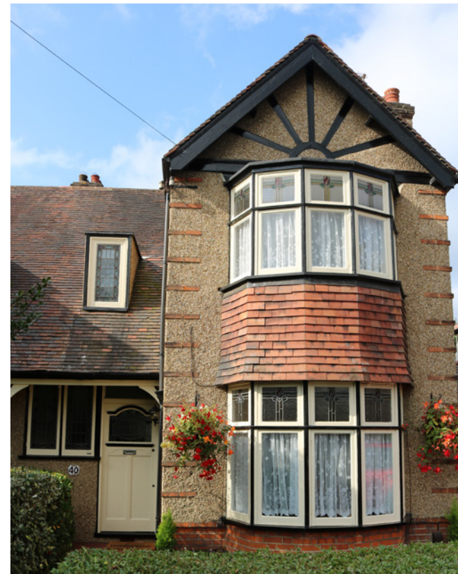
Intact timber window arrangement, Crossways
