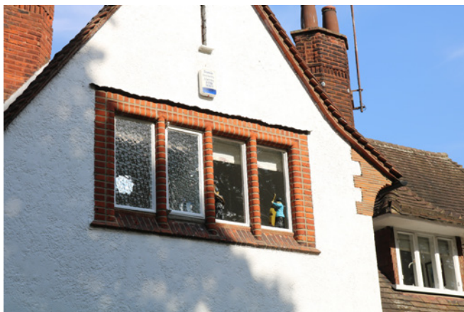
Horizontal window arrangement with brick mullions, Parkway
