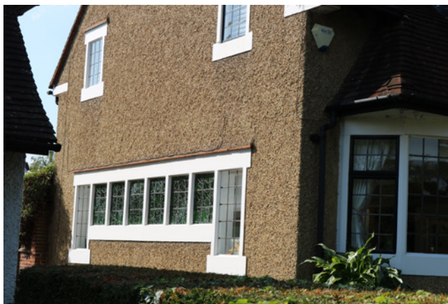
Decorative window to return elevation, Heath Drive
