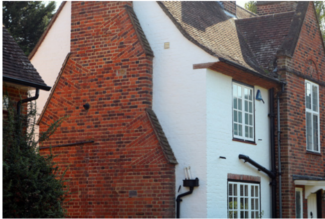
Detail of chimney brickwork.
