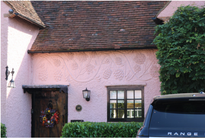
Detail of front elevation plasterwork.
