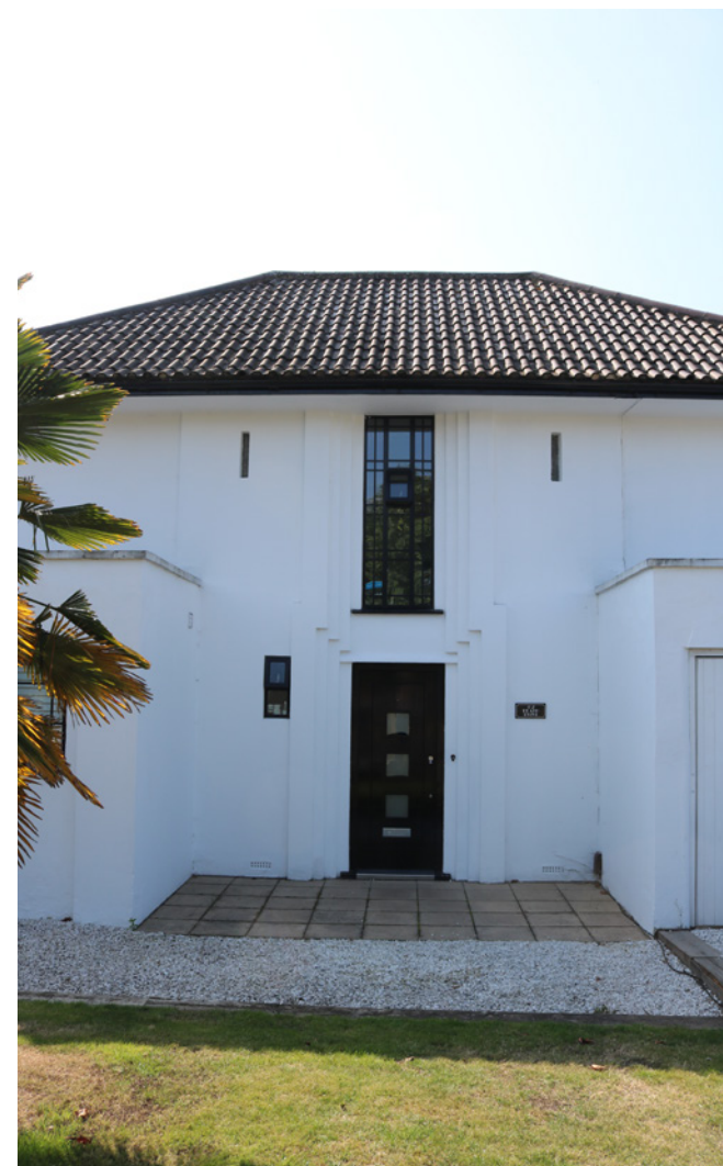
1930s front elevation detailing, Heath Drive
